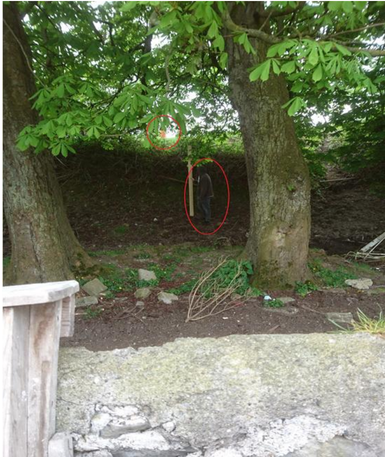
Image 1 Illustrates the significant height difference between the land at CELBRIDGE ROAD EAST (see traffic cone) and the ground level in the adjoining estate Leixlip Park. The traffic cone on CELBRIDGE ROAD EAST site is a metre above the man's (height 1.8m) head.
